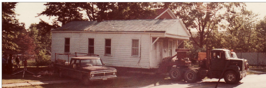
The tollhouse being backed into its current location.
