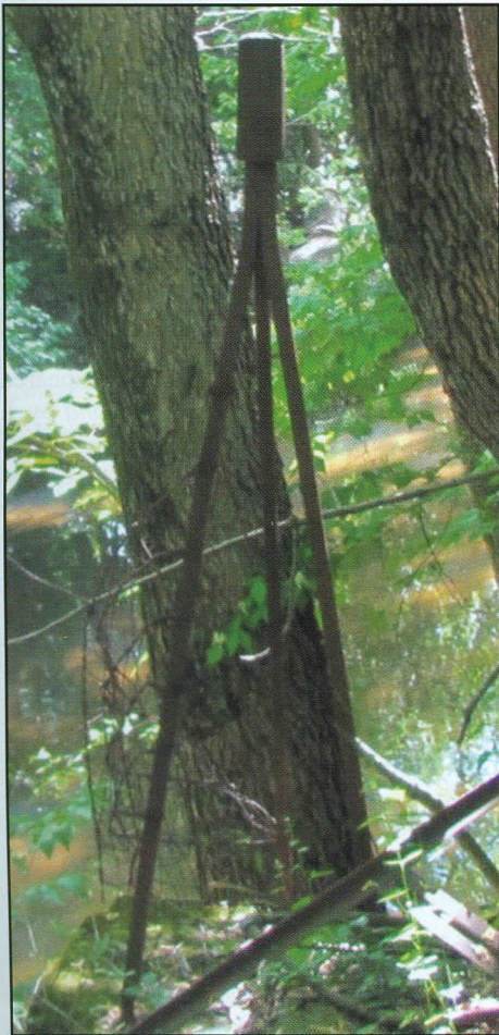
The wrought iron tripod with \frac{7}{8} " square legs and with a forged cable saddle is firmly anchored into the stone of the bridge abutment of William Lane's suspension bridge.
