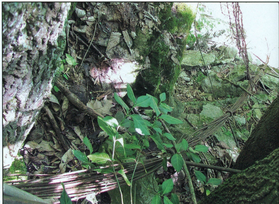
Look carefully to see the stranded suspension cable with the attached suspender irons, which nature has almost reclaimed, lying beside the stone bridge abutment.
