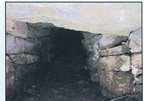
Puzzled by a port 7' down the side wall of the surface well just behind the Lane house, Lee snapped a picture for further investigation. To our surprise, we discovered a channel leading away from the surface well. Over time, a portion of the passageway has collapsed as shown by the debris in the channel. Our curiosity was definitely piqued! Bruce Whitteberry, assistant superintendent and hydrogeologist for the Greater Cincinnati Water Works, suggested we investigate the possibility of a conveyance system by looking near the water well for a natural spring well that could have manmade channels leading to ports in cisterns within both the residential structure and the smithy. As Whitteberry explained, the port that we had observed in the water well could have admitted spring water from nearby.
