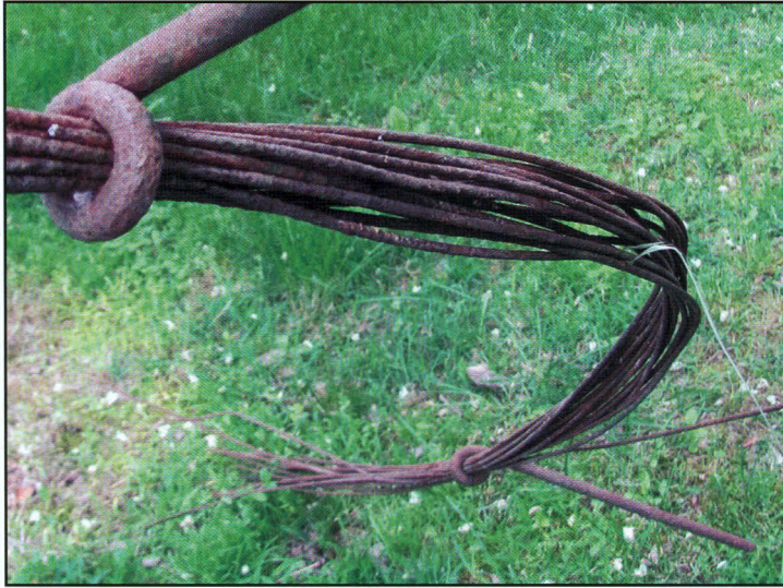
Here are the wrought iron suspenders that were forged around the \frac{3}{4} " diameter bundle of 18 strands of Number 8 wire laced straight (not twisted in the traditional wire rope configuration still used today). There may have been a single spiral wire wrapped around the bundle to maintain a cable configuration.
