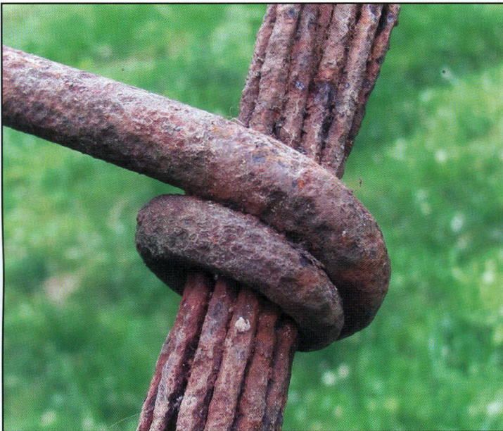
This iron suspender tightly surrounds the 18-wire cable bundle. Note the tapered end of the suspender iron as it snakes around the cable.
