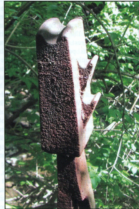
The wrought iron cable saddle was forged to the top of the iron tripod and features dual side saddles.
